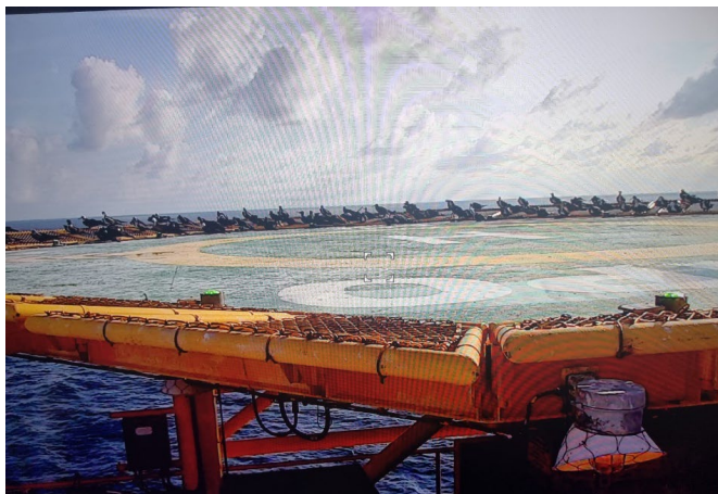
Figure 1 Typical example of bird roosting, clustered to the edges of helidecks that overlook the ocean.
