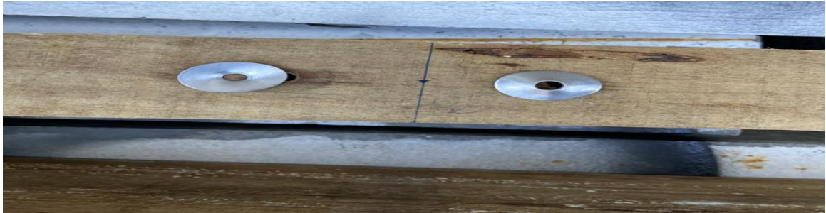
Figure 4 Bending of washers and indentation of the timber.
