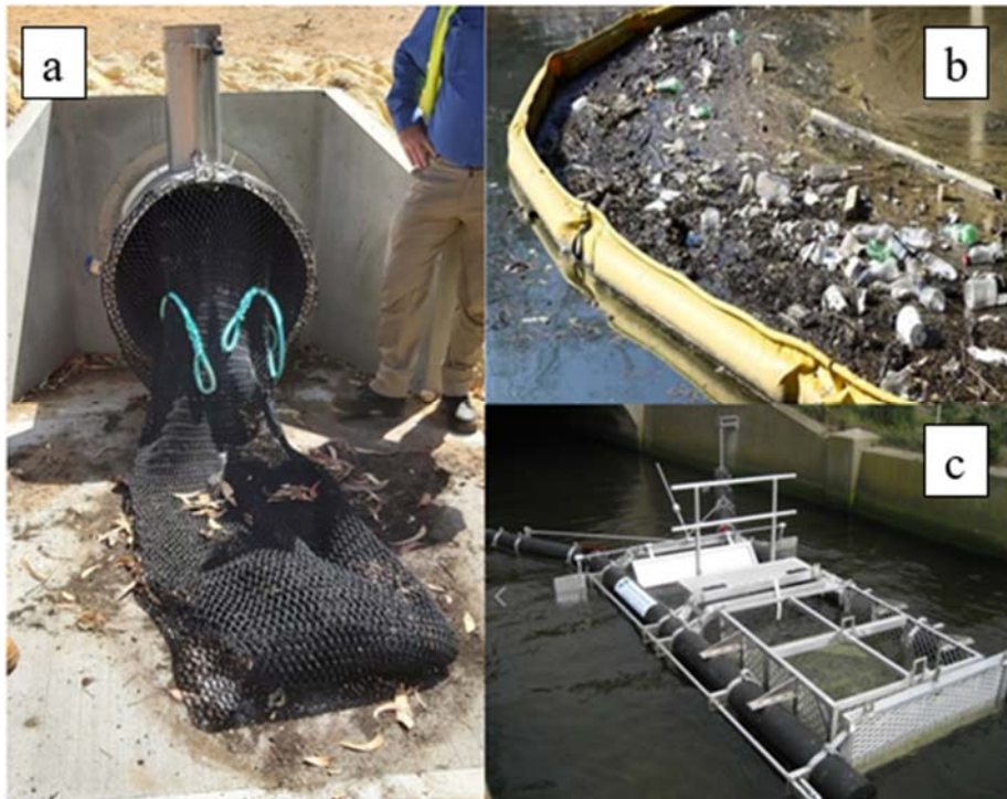
Figure 1 GPTs of interest: drainage net (a), floating litter boom (b), floating litter trap (c)
