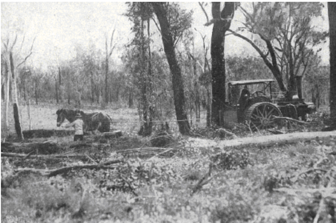
Figure 1 Perth to Albany Road 1927: Horse and steam tree-puller in preparation of the two-lane undivided highway (Main Roads WA 1927)
