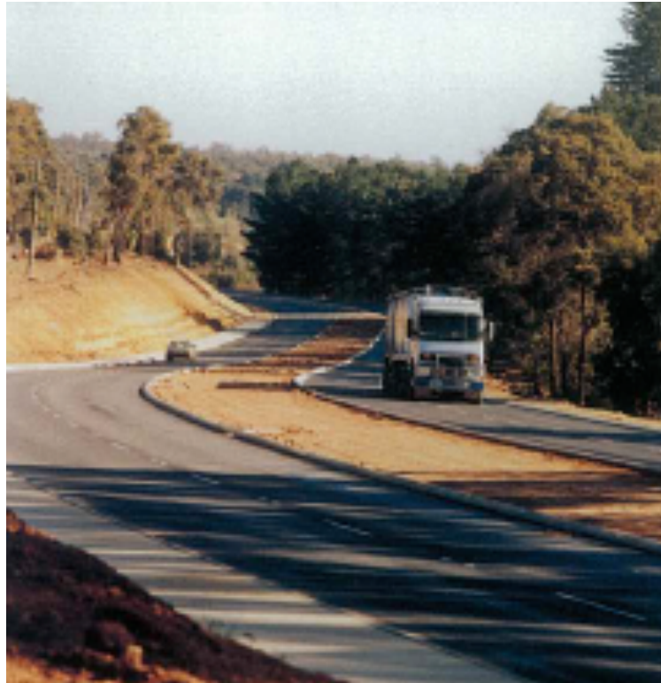
Figure 2 The Albany Highway 1999: Reconstruction of section involved the improvement of 23 curves and construction of a four-lane divided carriageway on Bedfordale Hill (Main Roads WA 1999).
