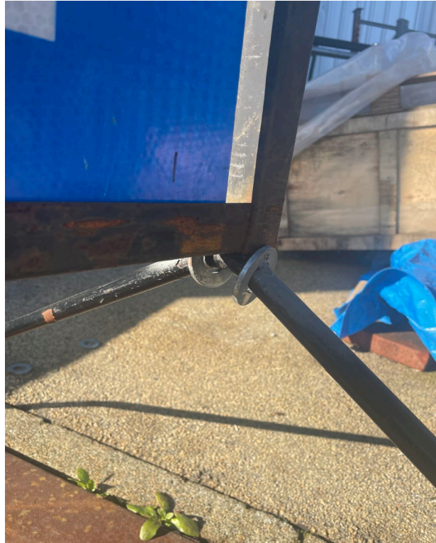
Figure 3 The welded washer approach installed in the field
