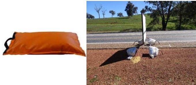
Figure 1 Sandbags and how they are used (Main Roads Western Australia, 2020)
