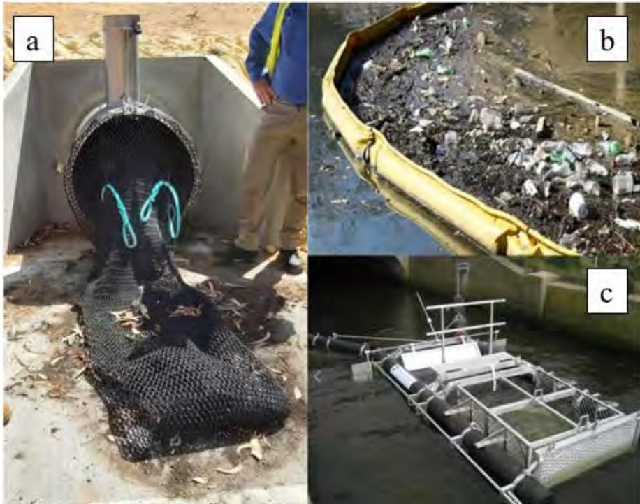
**Figure 1** GPTs of interest: (a) drainage net, (b) floating litter boom, (c) floating litter trap.
