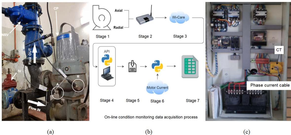
**Figure 2** Accelerometers in Axial “A” and Radial “R” directions, Non-return Valve as “NRV”, Isolation Valve as “IV” and Centrifugal Pump as “CP” shown in (a). Data management schematic diagram shown in (b) and installation of current transformers “CT” inside the control panel of pump stations to measure motor current shown in (c).
