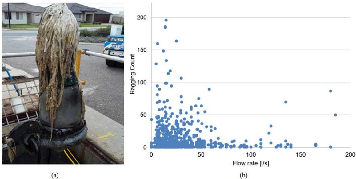
**Figure 1** Rags caught on pump body at a WWPS, Perth shown in (a). Ragging count from January 2016 to December 2019 shown in (b) where each dot represents a WWPS.
