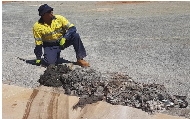
Figure 1 Figure 1. Water Corporation mechanical tradesperson next to a 2m Obstruction, removed from a West Australian sewer, 2017. [Dougherty, The West Australian , 2017]
