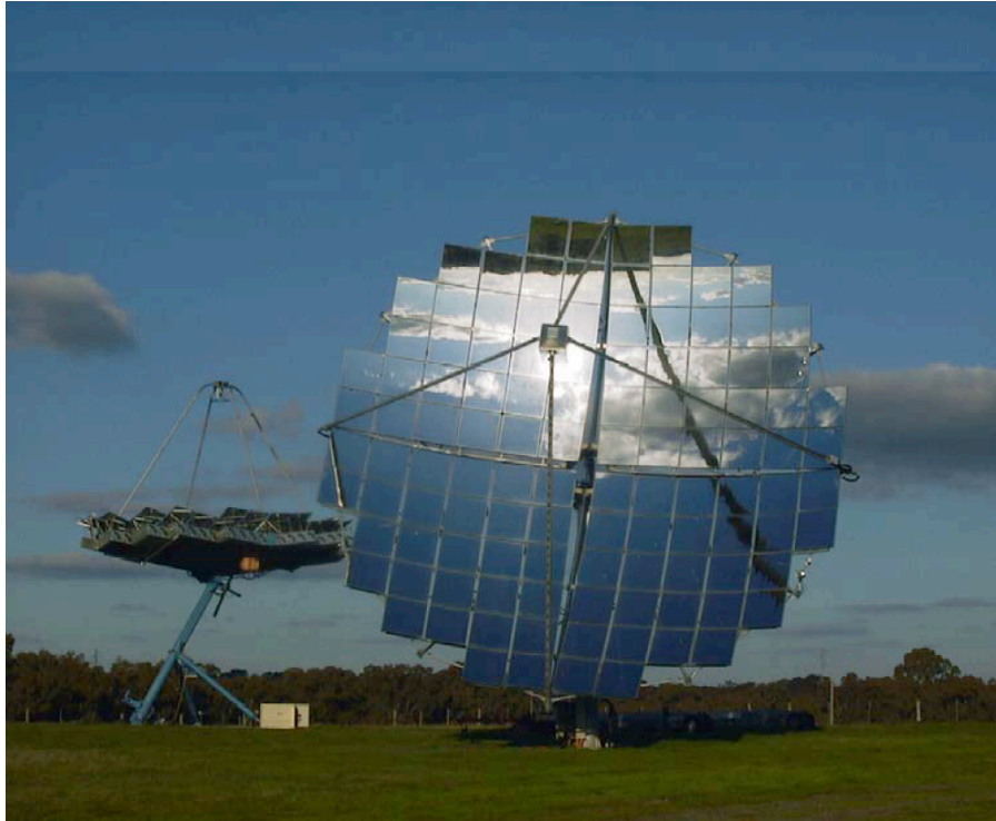
Figure 1 CS-500 parabolic dish collector by Solar Systems based near Bendigo, Victoria
